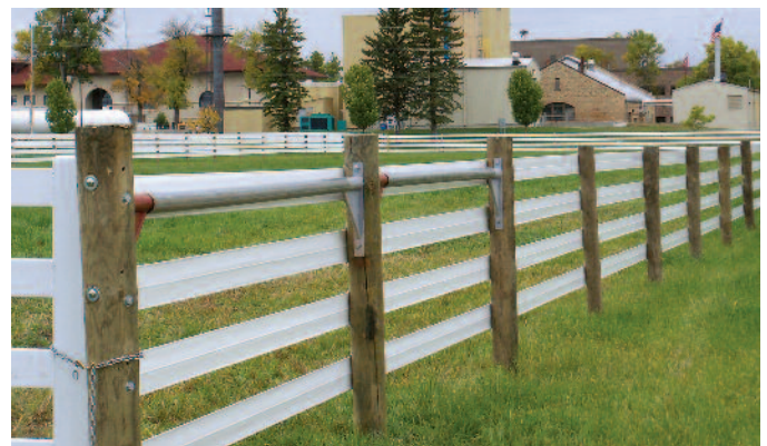
The University of Minnesota's Equine Center uses flat ribbon fencing and 5" wood posts to provide a safe and sturdy enclosure.
