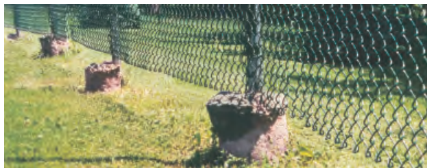
A striking, but not unusual, example of frost-heaving
