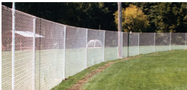
Drive Anchors and hi-tensile wires serve as bracing for a "topless" chainlink fence.
